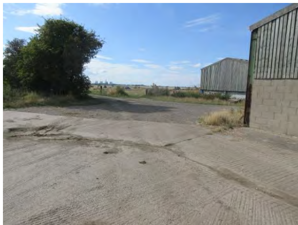
Photograph 15. Farm access through outbuildings. Load moves away from camera. Negotiable with caution and with courtyard kept free of vehicles and any other items that could be in store. Note there is a gradient here and change of level but this is negotiable by using trailer hydraulics.
